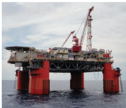
Moored in MC 547, LLOG Exploration's Who Dat field semisubmersible production unit, OPTI-EX, has 60,000-b/d, 150-MMcf/d oil and gas handling capacity. Photo courtesy LLOG.
